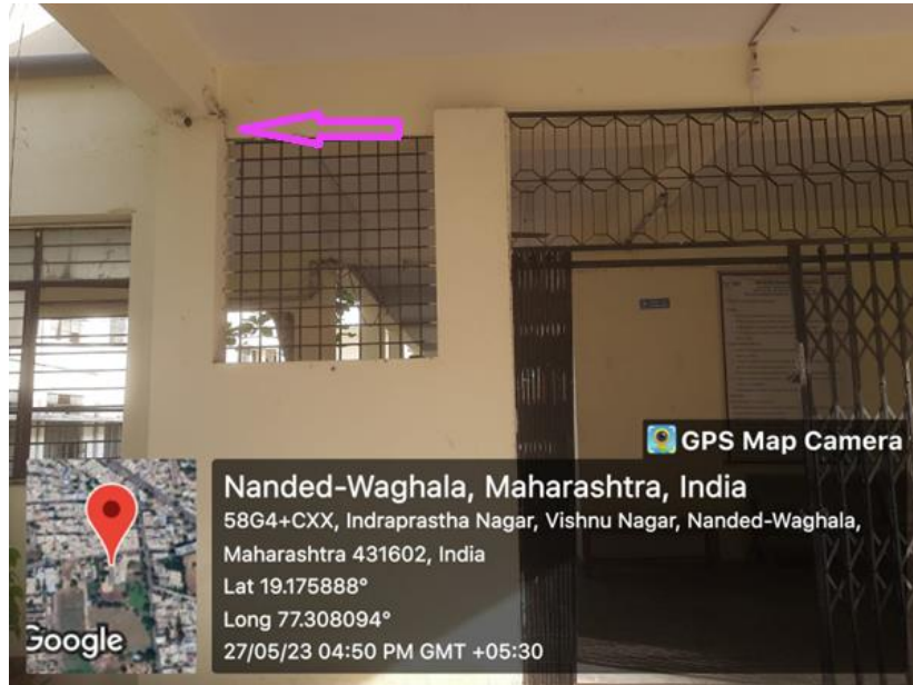
CCTV CAMERA AT ENTRANCE
